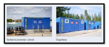
is the use of prefab solutions from containers. This method involves using shipping containers as building blocks to construct various infrastructure and superstructure facilities, including offices, restrooms, storage areas, and other supporting structures. Prefabricated container solutions can be designed and assembled off-site, reducing construction time and costs while ensuring quality control.
