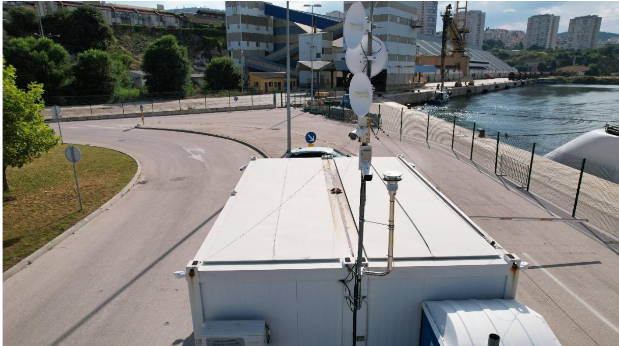
Figure 16. Land sensors for receiving information from buoys 2 (photo made by air drone)
